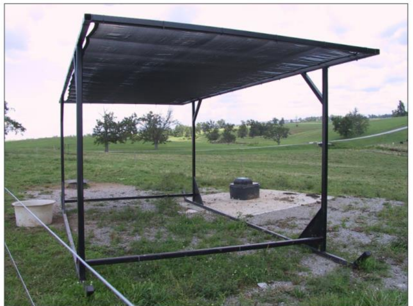
Figure 2. This shade structure is portable, so it can be moved with the animals. It has a shade cloth roof.
